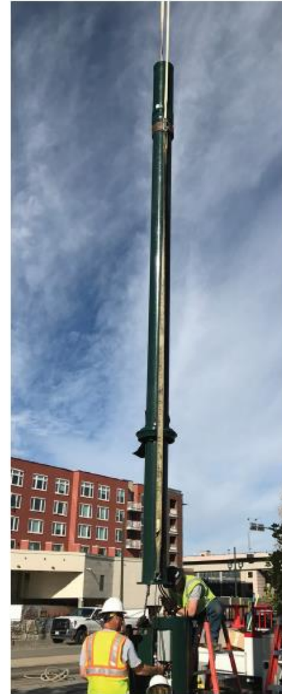
Step 3: Install top section with antenna onto base section with architectural shrouds.
