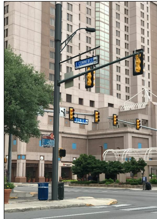
CityPole Traffic Signal Reduced Footprint in ROW
