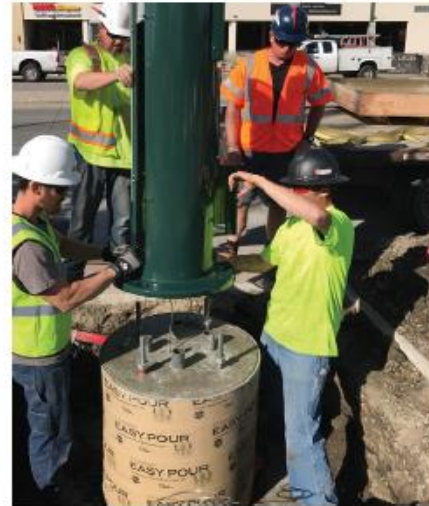
Step 2: Install base cabinet of the CityPole® onto the foundation and secure
