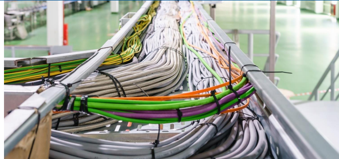
Multiple layers of single-purpose infrastructure
