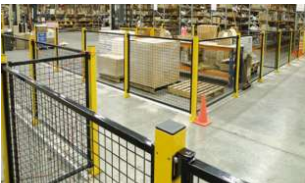
Machine Fencing Guard
