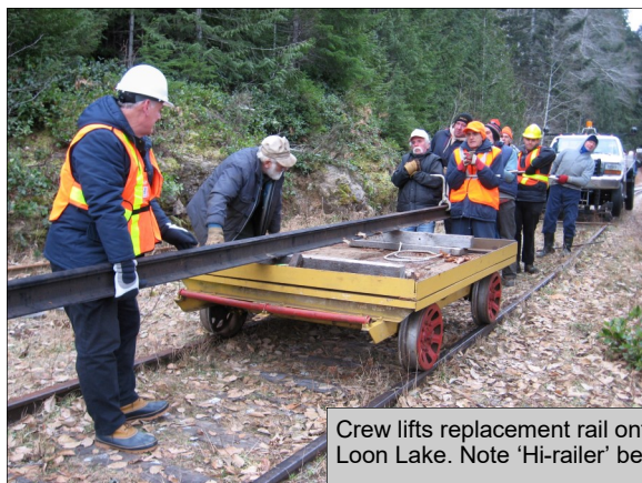
Replacement rail rolled into place Note fallen tree trunk beside track
