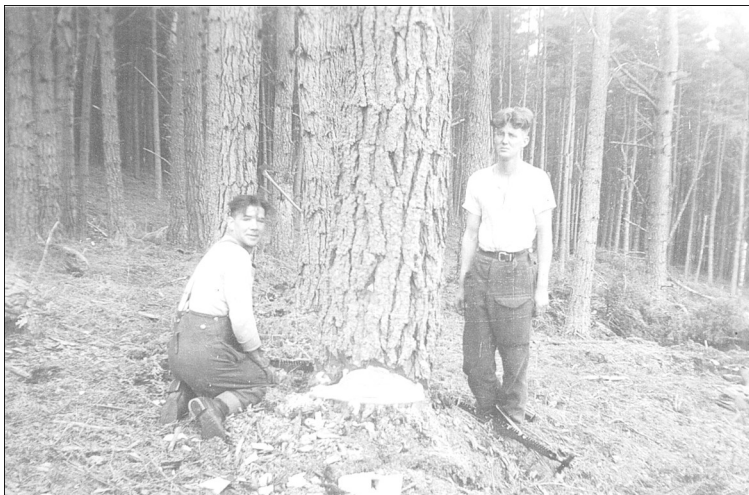
Putting in the Undercut Note how low it is to the ground. Note also the crosscut saw laying in front. There were some Douglas fir plantations but pine, spruce and larch were the main species logged.
