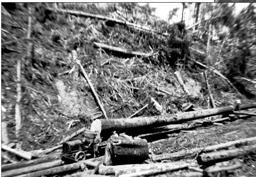
“Fore-and-aft” Road in Quatsino Sound made of hewn timbers laid on log cribbing to create a level hauling road.
