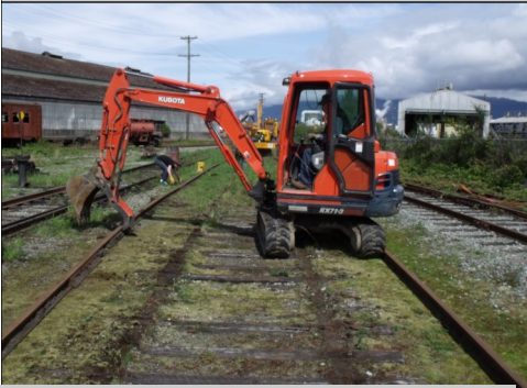
(above) Ken Fyfe lifts rails (still connected) to the side, to expose rotten ties.
