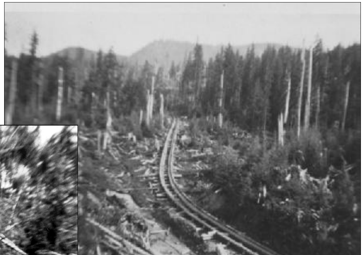
“Fore-and-aft” Road in Quatsino Sound made of hewn timbers laid on log cribbing to create a level hauling road.
