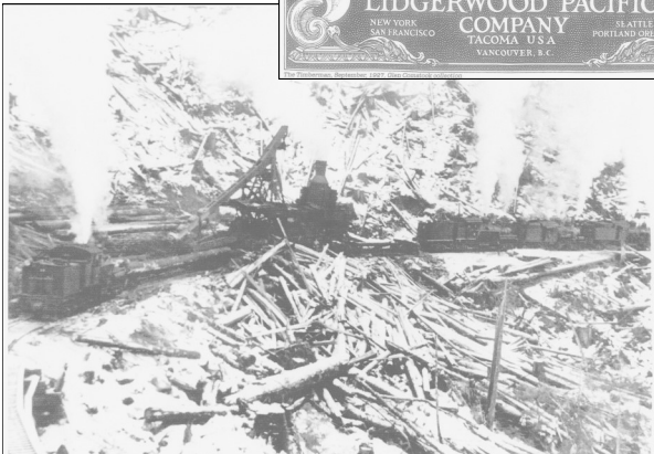
"Lidgerwood" derailed (1945) "YO-3" derailed while moving to a new setting at Franklin River. It took 4 locomotives to put it back on track: a 90-ton "Shay", a 70-ton "Shay", a 50-ton 'Climax' and a 60-ton "Shay".
