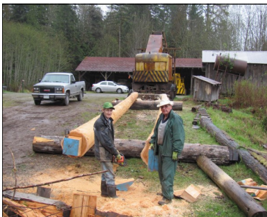
REBUILDING THE A-FRAME "J.J." inspecting Ron Green's work.
