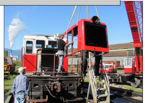
(above) Lowering hood into place
