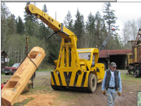
Swinging the base log into position
