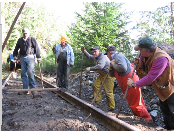
(above) Ken Fyfe knocks down broom with his flail mower, much to the joy of the rest of the crew. Photo: Sterling Stump (below) Crew levers rail into place at rockfall site. Rob Gair (l.) checks track gauge while crew (l. to r.) N. Malbon, P. Geddes, L. Evans & R. Clark lever the rail.
