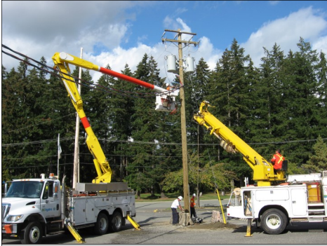
B.C. Hydro crews connect new line to the I.H.C.
