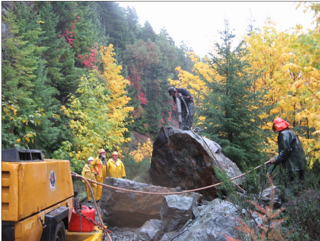
(above) Breaking up the Big Rock Steve Middelkoop operates the hydraulic rock splitter. (below) The ‘Landscaper’ prepares to park for the night. Other photos: D. Hooper
