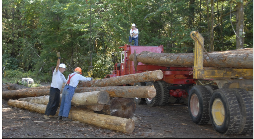
SOUP'S LATEST ERECTION lifting tank onto the water-tower at McLean Mill.
