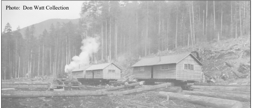
Three Bunkhouses being 'spotted' by the loci before unloading. Note the logs at right angles, ready to be used to slide buildings into place. A 'Cat' is ready to the left, to pull the bunkhouse off the skeleton car.
