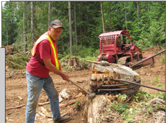
(below) Tony spiking a guy line to stump
