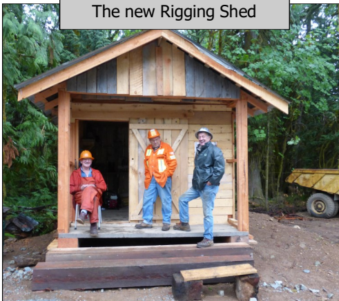
The new Rigging Shed
