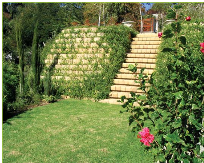
4x4 STEP BLOCK STAIRS AND HEAVY GRAVITY RETAINING
