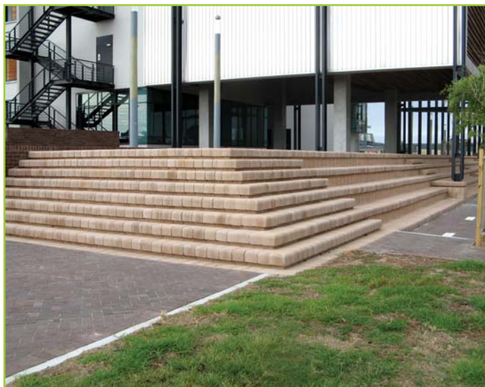
SEATING AND STEPS - 4x4 BLOCKS AND L12 BLOCKS
