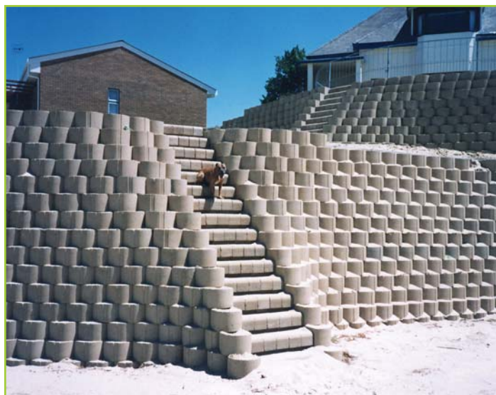
INSTALLATION READY FOR LANDSCAPING
