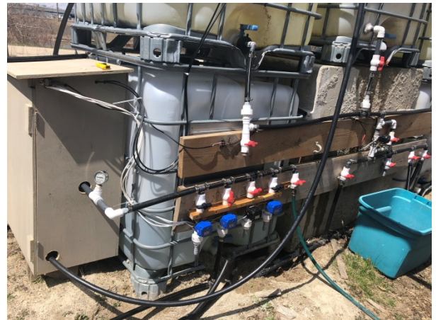
Solar powered pumps, valves and timers for irrigation circuits
