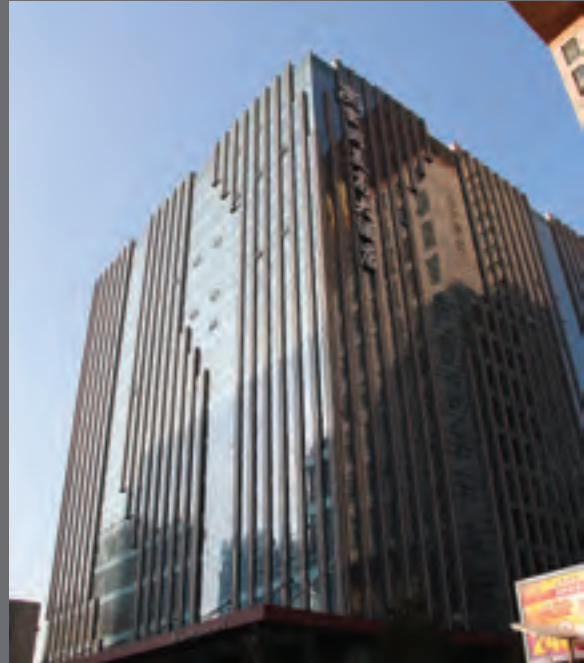
Hotel of Shanxi Prestigious hotel in the center of the mountain town of Shanxi, furnished with Orbis washbasins and Sa.02 and Kimi sanitary wares.
