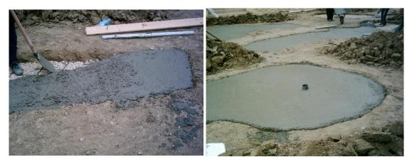
4. **The frame of natural cement** (half sand, half cement) will be poured in special molds of structural iron. They are reinforced in the upper part by means of steel rods, diameter 6 mm, and accurately connected to the slab. For this purpose, the borders of the slab are not concreted at the same time as the main part and the ends of the upper reinforcement are curved up 5 cm. In distances of 2 m, drain openings of the appropriate size are provided for.
