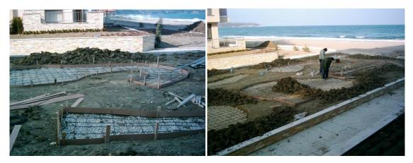
3. The reinforced slab, which constitutes the actual fairway, will be poured in forms using Portland concrete ( $300 \text{ kg/m}^3$ ). Thickness will be 10 cm. The surface of the layer must be absolutely horizontal for all fairways or parts thereof. The surface of the slab will remain as rough as possible in order to warrant secure resting of the layer (of colored concrete).
