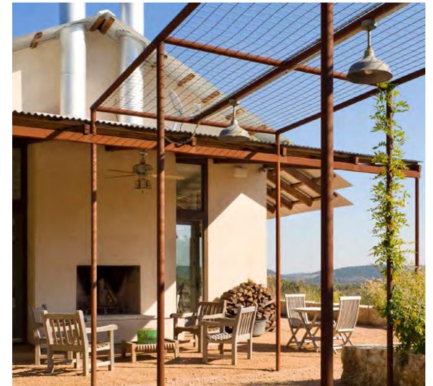
locally sourced materials are selected for their richness, low maintenance and practicality to help the buildings blend into the environment.
